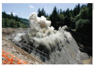
Explosives blast the first cracks in Marmot Dam July 24.
